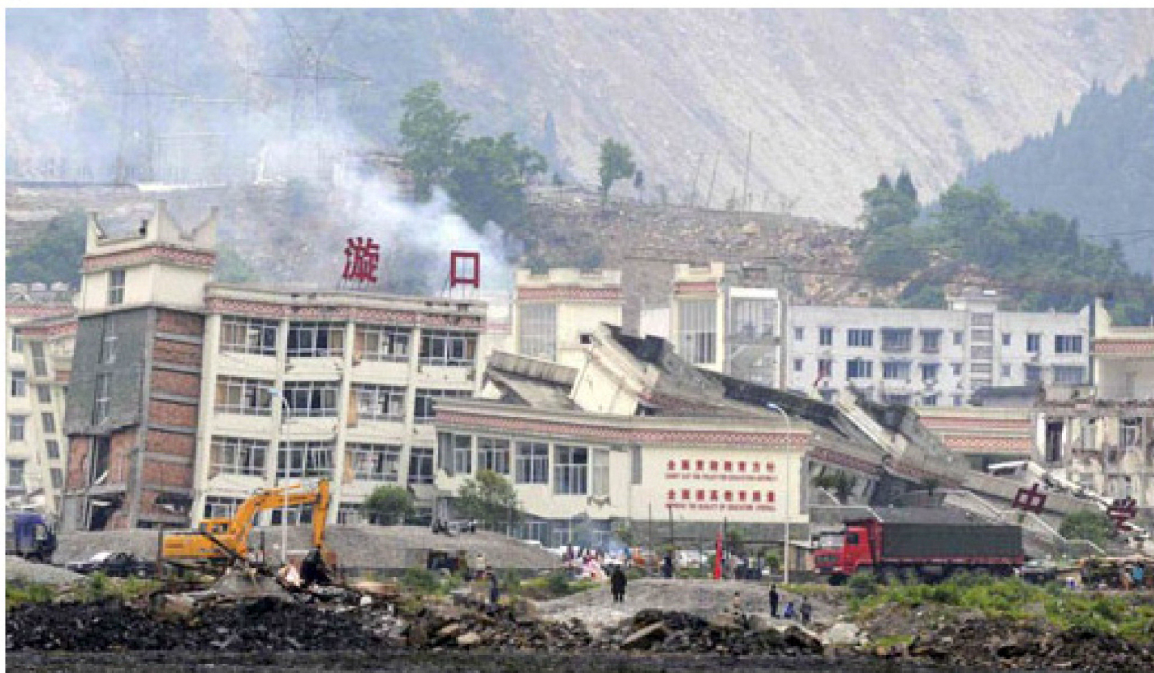
A collapsed school in Wenchuan county. Photograph: Reuters
