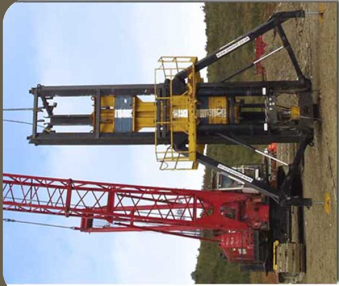
3MN STATNOMIC Load Test
